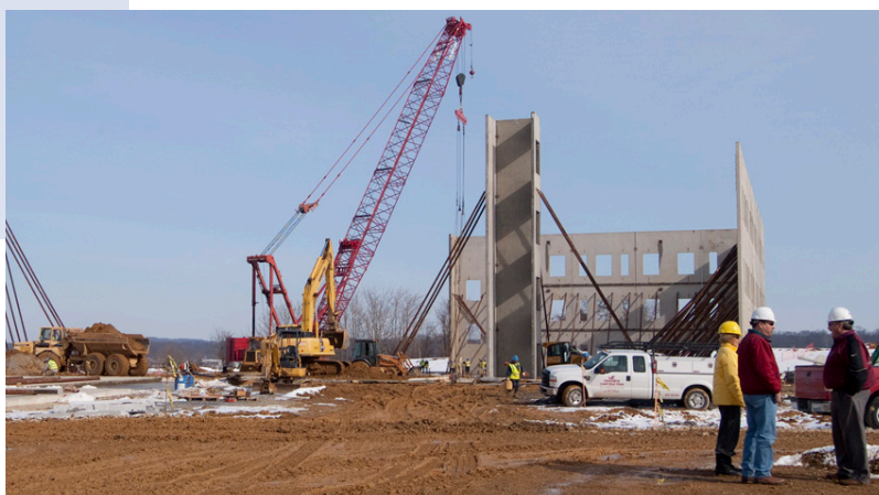
The panel is set into place.
