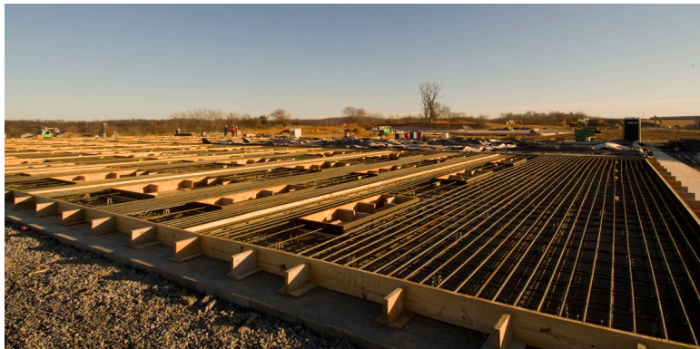
The walls are made from giant precast concrete panels.
