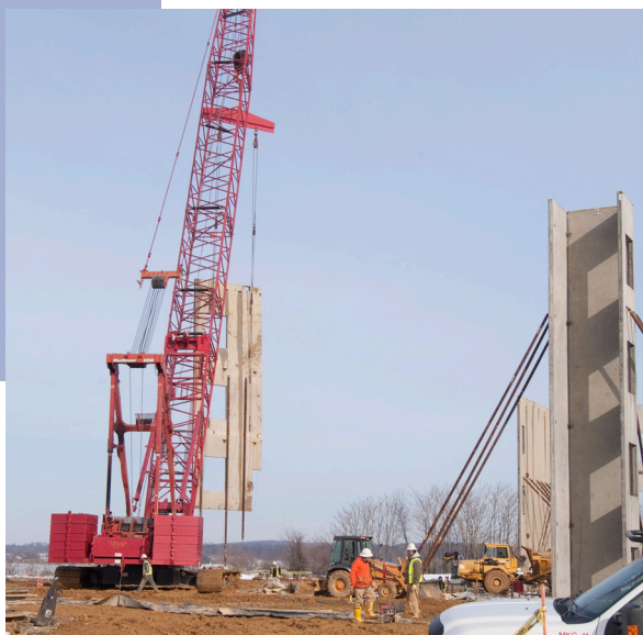
A panel is lifted by the crane and moved into position.
